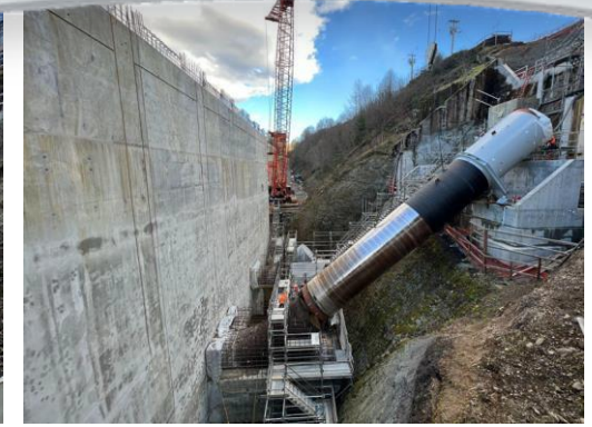
Penstock installed and ready to be connected to the dam.
