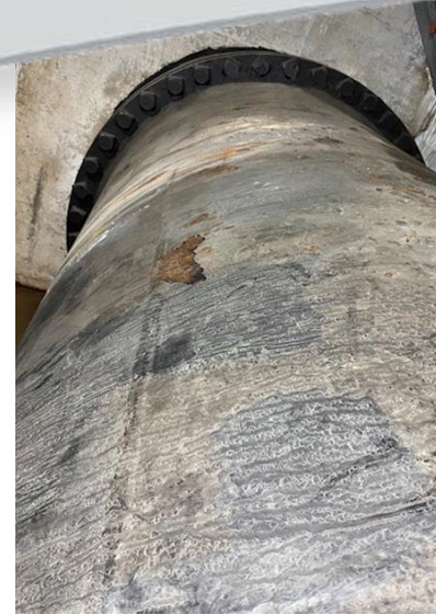
The existing coating had begun to peel and flake, revealing the lead paint system underneath.
