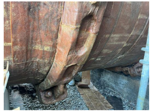
Close up of the irregular clamps coated with Temcoat™ 3000 primer and Wax-Tape® #1 wrap.
