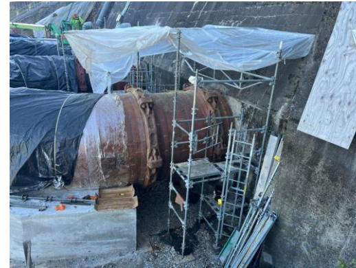
Settlement and Victaulic joint wrapped with Temcoat™ 3000 primer and Wax-Tape® #1 wrap.
