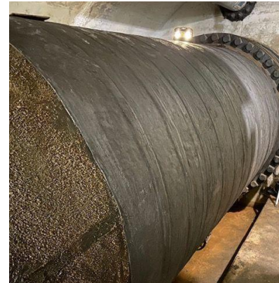
The existing coating had begun to peel and flake, revealing the lead paint system underneath.
