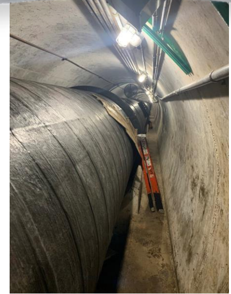
Temcoat™ 3000 primer and Wax-Tape® #2 wrap (black) were applied to 54' of the 280' penstock. This will be repeated each year until the penstocks are completely coated.
