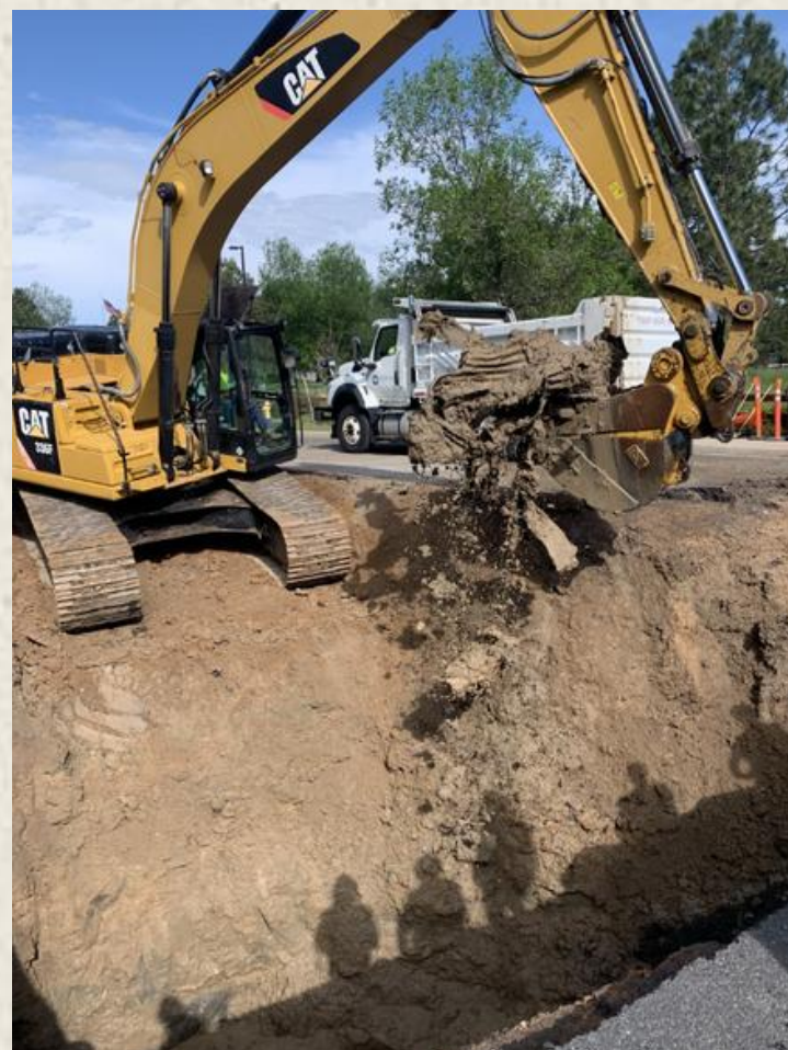
Infrastructure Installation & Repairs
